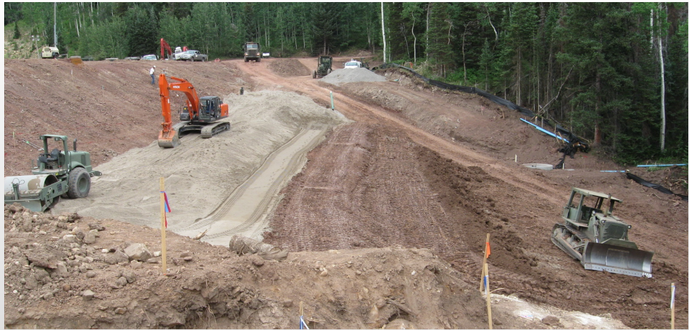
Reservoir #1 Dam Reconstruction
