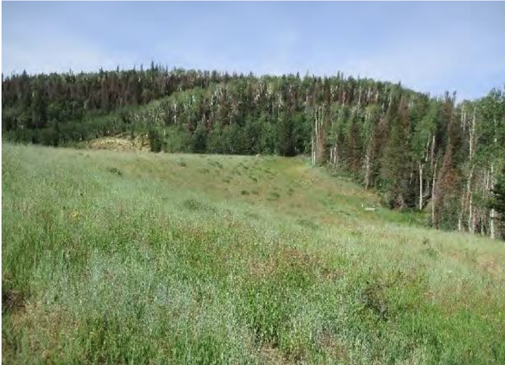
View of the downstream slope taken from the right abutment.
