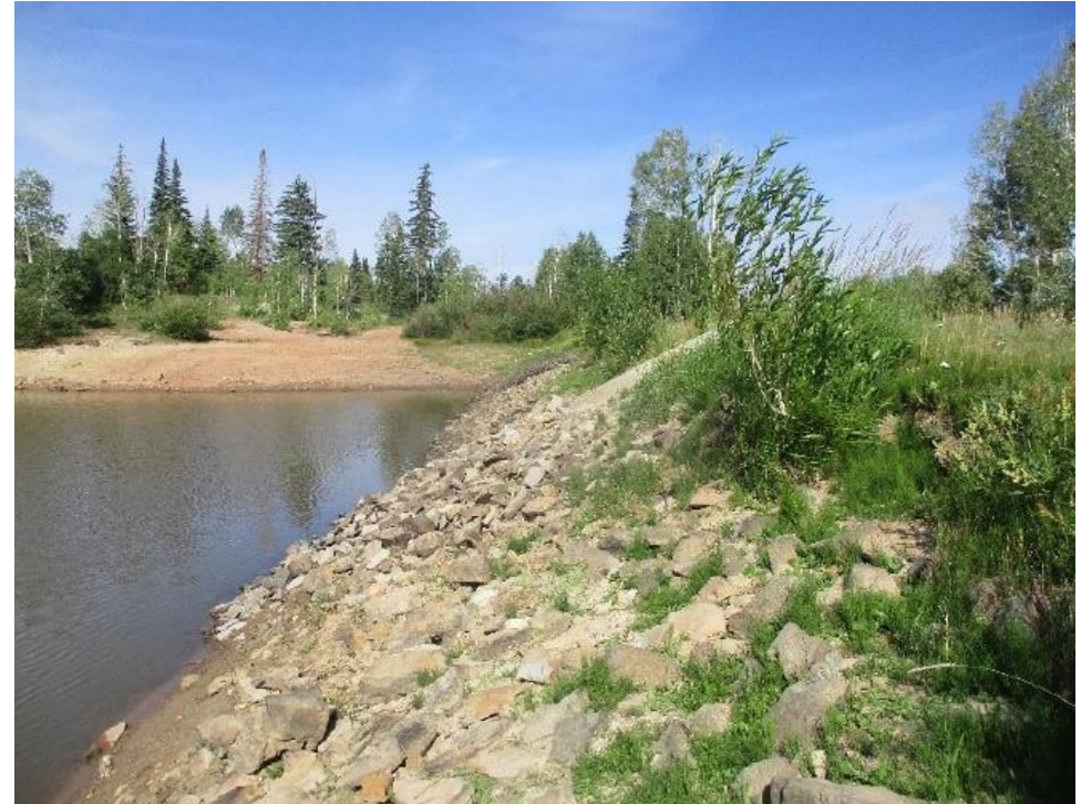
Looking across the upstream slope from the right abutment.
