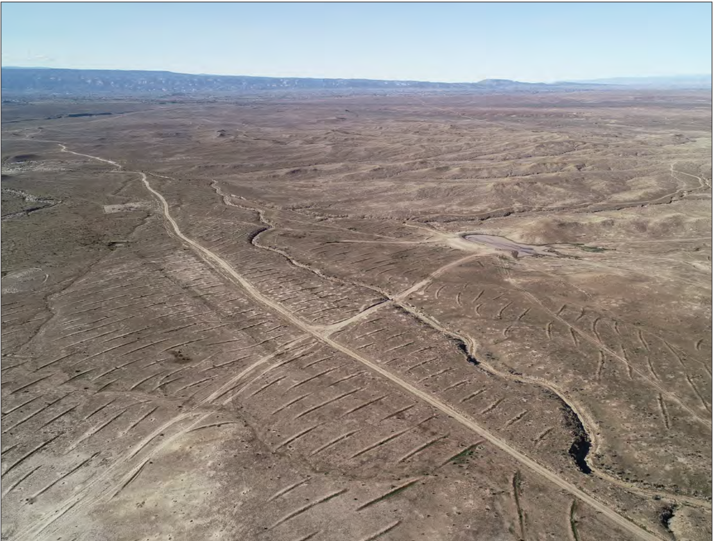
Terracing for erosion control
