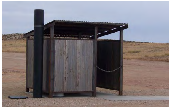
“Moab style” steel vault toilet structure
