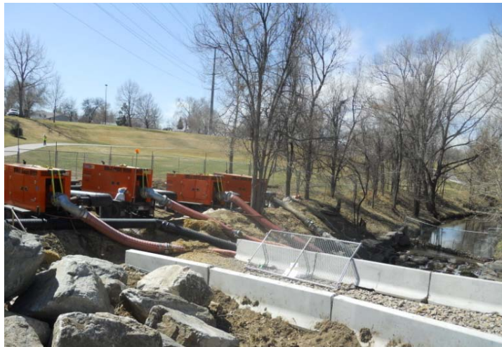
Photograph TDM-2. Despite a relatively significant baseflow, a pumped diversion was selected for this Lakewood Gulch project due to a lack of space crossing Federal Boulevard. Photo courtesy of City and County of Denver.
