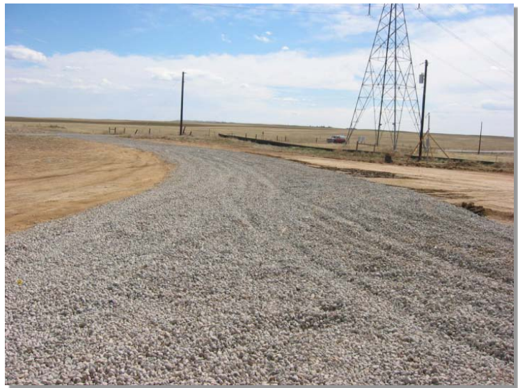
Photograph SCR-1. Stabilized construction roadway.
