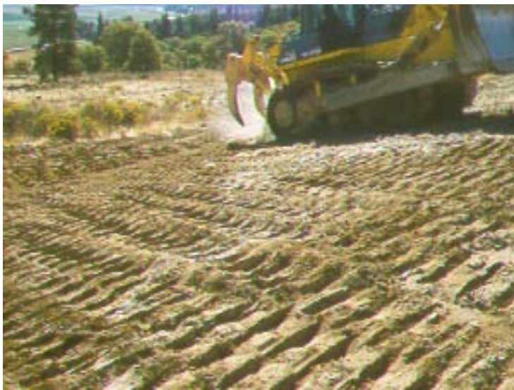
Photograph SR-1. Surface roughening via imprinting for temporary stabilization.
