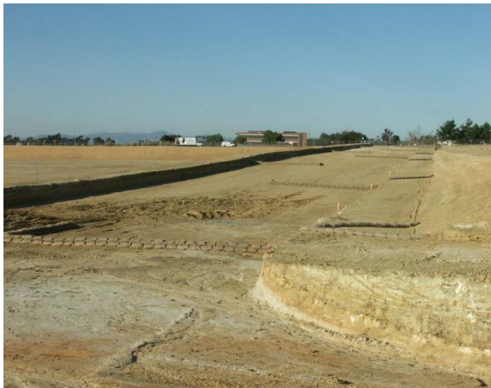
Photograph RCS-1. Rough cut street controls.
