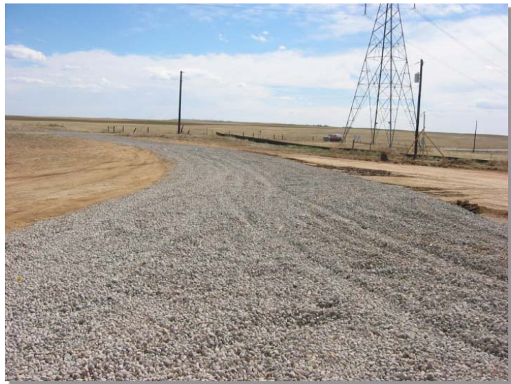
Photograph SCR-1. Stabilized construction roadway.
