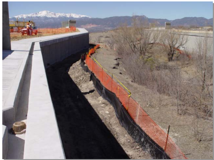
Photograph PV-1. Protection of existing vegetation and a sensitive area. Photo courtesy of CDOT.
