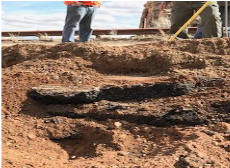
Road Construction – Pavement Layers March 19, 2018
