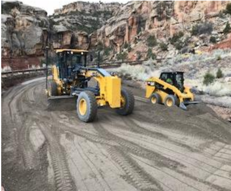
Construction Below the Tunnel March 20, 2018
